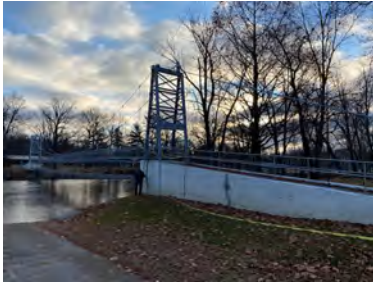
Starting to measure on a dark morning in November.
